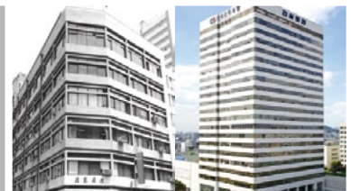
1963.07. Proclamation of the Construction Guarantee Act
